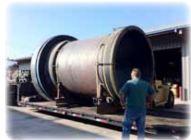
This "spool" for 108" pipe was lowered into a vertical pipe at the bottom of a surcharge tower that could not have the flow shut down. Grout was then pumped into the void between the end bladders to fill up and block off an intersecting horizontal pipe. The "spool" was left in place.
